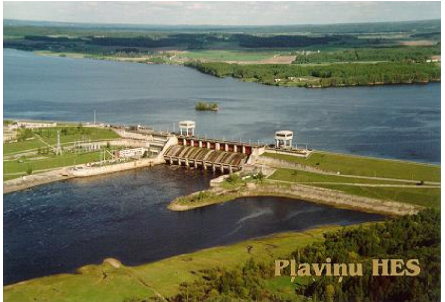
Above : Plavinas Dam (70 m height): The main power station in Republic of Latvia
