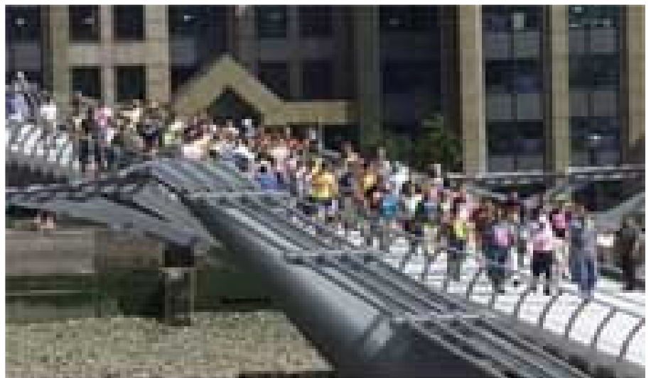
Above : Loading test with 120 people
